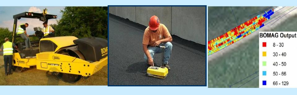
Current IC technology is accelerometer-based.
