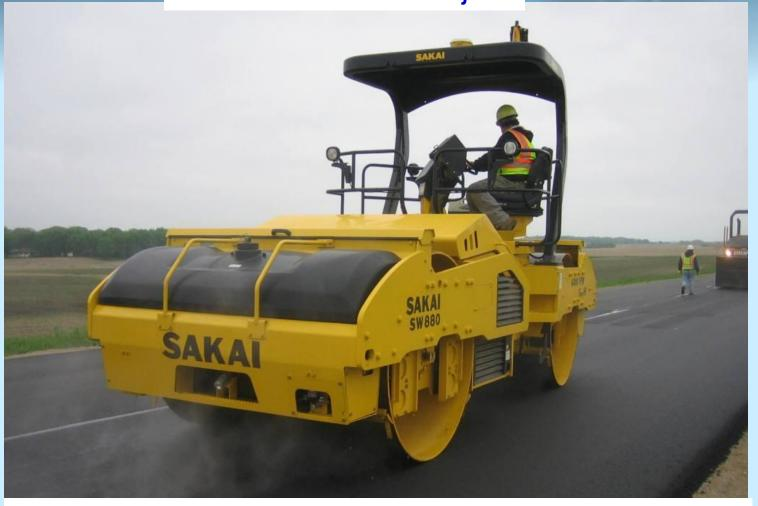
Compaction/mapping of HMA base course layer
