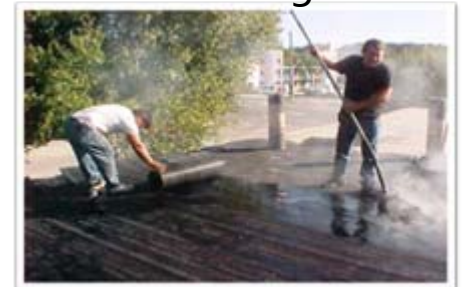
Built-up Asphalt Roofing
