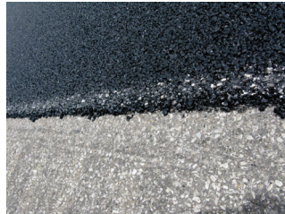
Aggregate Breakage Due to a Roller
